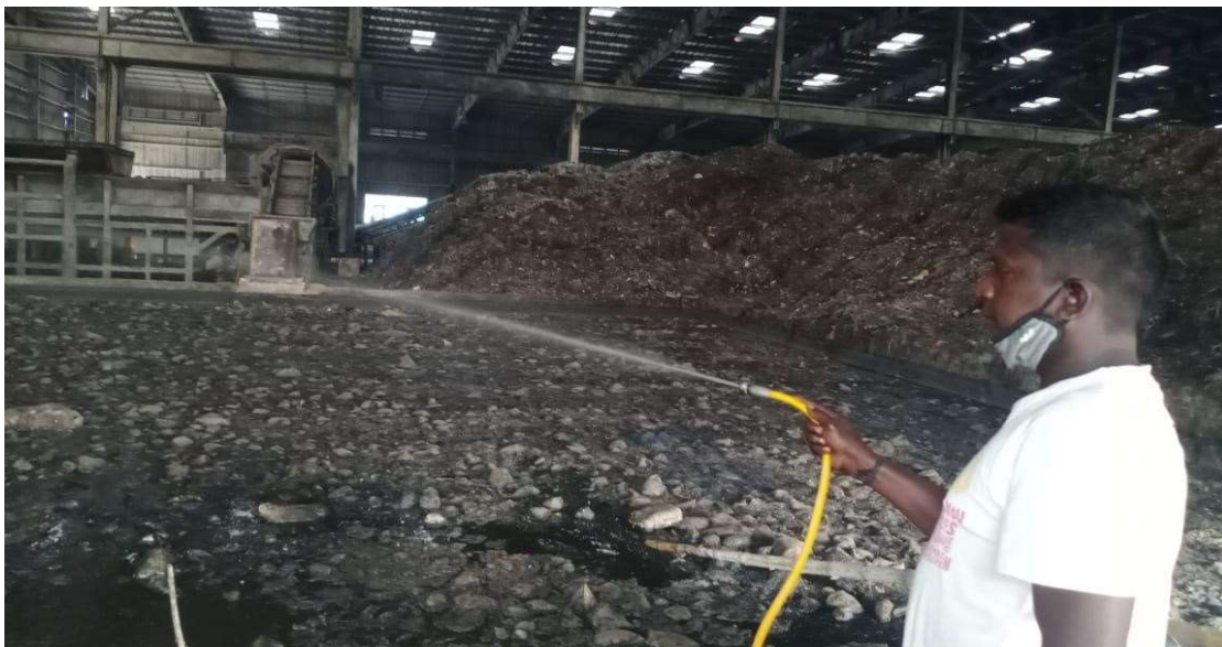
Figure 2 Leachate Treatment spray
